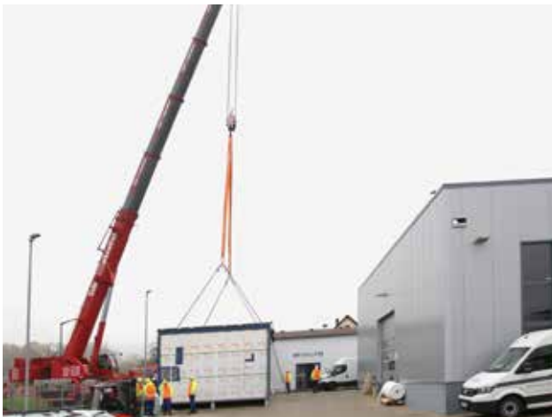
Fast-Track facility in container design suitable for lifting with crane and transport with HGV or ship
