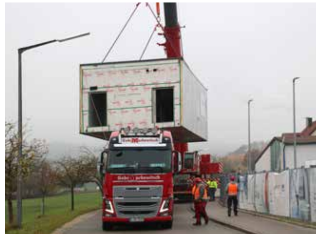
Fast-Track facility in container design suitable for lifting with crane and transport with HGV or ship
